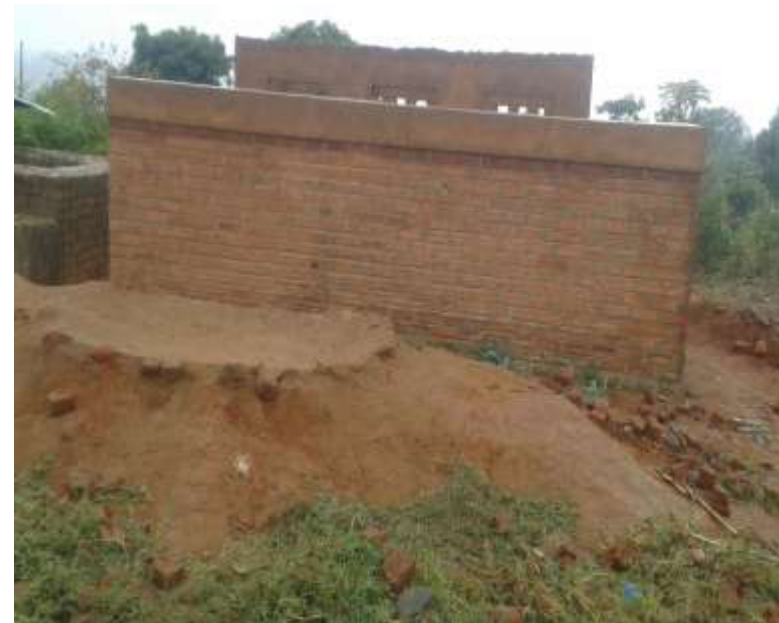
An uncompleted set of toilets in Thy
