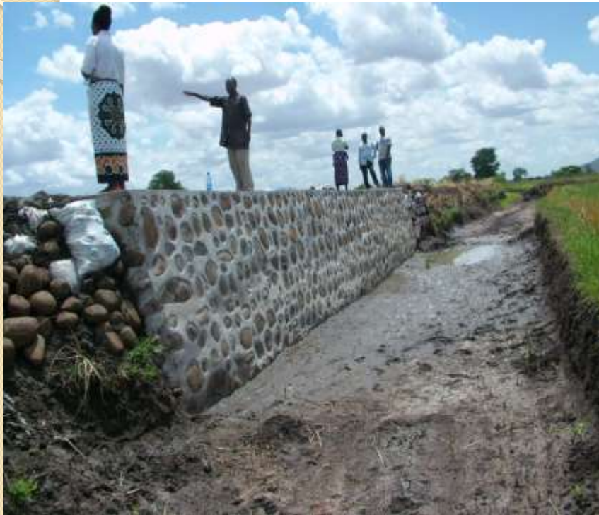
Dyke constructed by Tamani CBO in PE
