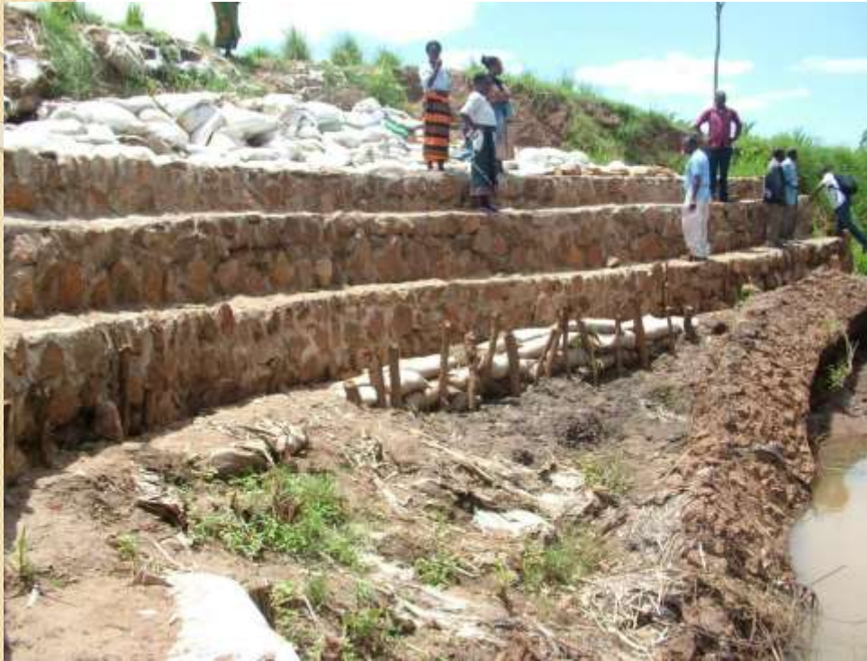
Dyke construction by Kanjedza CBO
